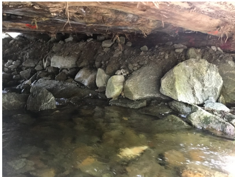
Right Bank Abutment when facing downstream
