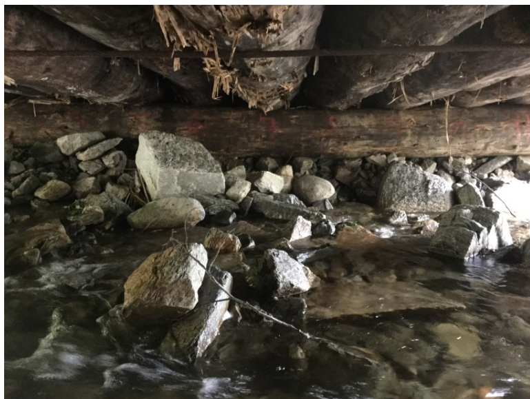
Left Bank Abutment when facing downstream
